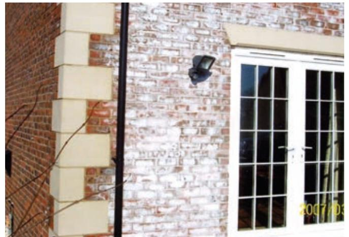
The first 3 to 5 days after laying (dependent on season), brickwork is most vulnerable to the elements as mortar is still undergoing the hardening process. Newly erected masonry should be covered by waterproof sheeting to protect fresh mortar and open cavities to stop masonry becoming saturated. Hessian is not waterproof. Once the structure is watertight, i.e. roof and windows in place, the building can commence the drying process.
