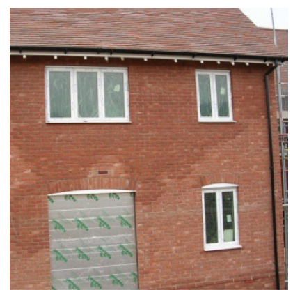
Saturation occurring prior to roof & window placement.
