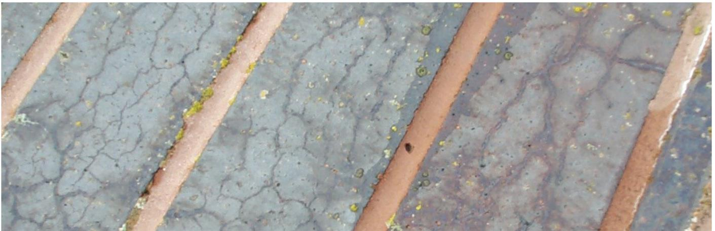
The effect of crazing is not uncommon to dense, strong wire-cut bricks especially if they have a smooth face finish. It is, however, far more noticeable on smooth blue types of brick.
